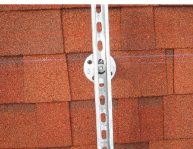
SAMPLE PHOTO : GALV. FLANGE W/ UNISTRUT P1000T
