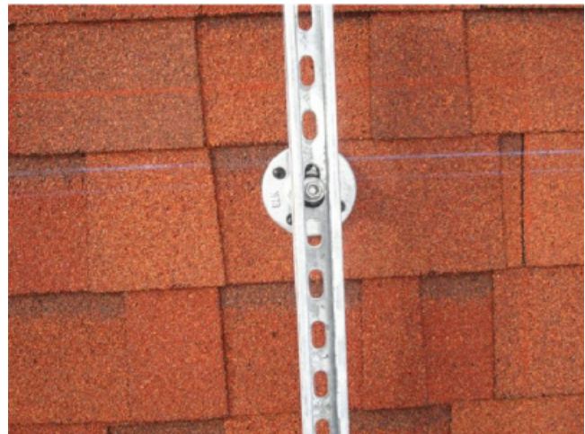
SAMPLE PHOTO : GALV. FLANGE W/ UNISTRUT P1000T
