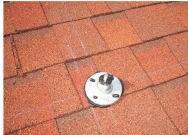
ONE-INCH PIPE NIPPLE AND GALVANIZED FLANGE SERVE DUAL-PURPOSE AS BOTH STRUCTURAL SUPPORT AND ROOF SEALANT FILLED PITCH-POCKET. CONTRACTOR SHALL FILL NIPPLE WITH PL1 OR EQUAL POLYURETHANE ROOF SEALANT AS SHOWN IN ADJACENT PHOTOS.
