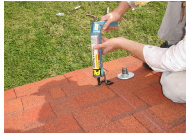
ONE-INCH PIPE NIPPLE AND GALVANIZED FLANGE SERVE DUAL-PURPOSE AS BOTH STRUCTURAL SUPPORT AND ROOF SEALANT FILLED PITCH-POCKET. CONTRACTOR SHALL FILL NIPPLE WITH PL1 OR EQUAL POLYURETHANE ROOF SEALANT AS SHOWN IN ADJACENT PHOTOS.
